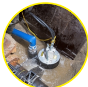
Underground Pipeline Maintenance
